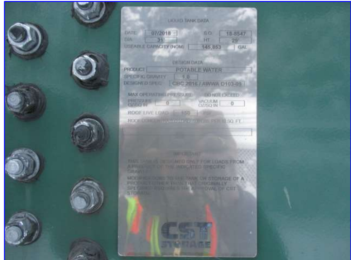
Photo 4 – Exterior (Jan 2020) – Tank manufacturer’s nameplate.
