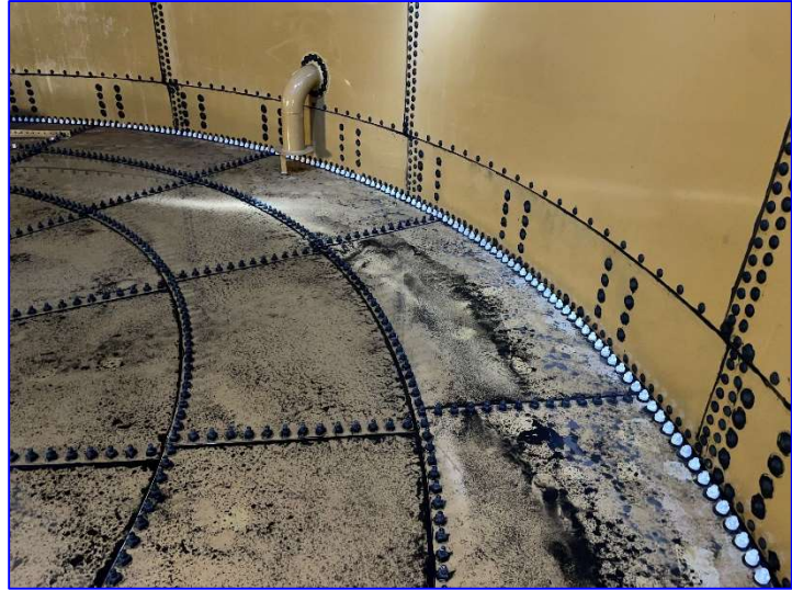
Photo 25 – Interior (June 2022) – Overview of the shell and tank bottom.
