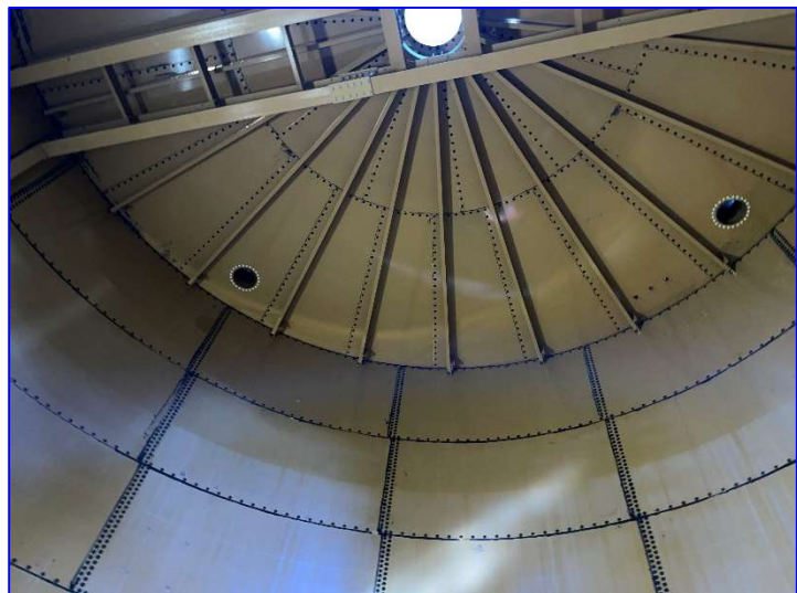
Photo 21 – Interior (June 2022) – View of the interior bridge supported roof structure.
