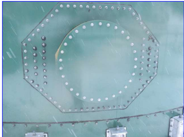
Photo 5 – Exterior (Jan 2020) – View of the tank shell manway (1 of 2)
