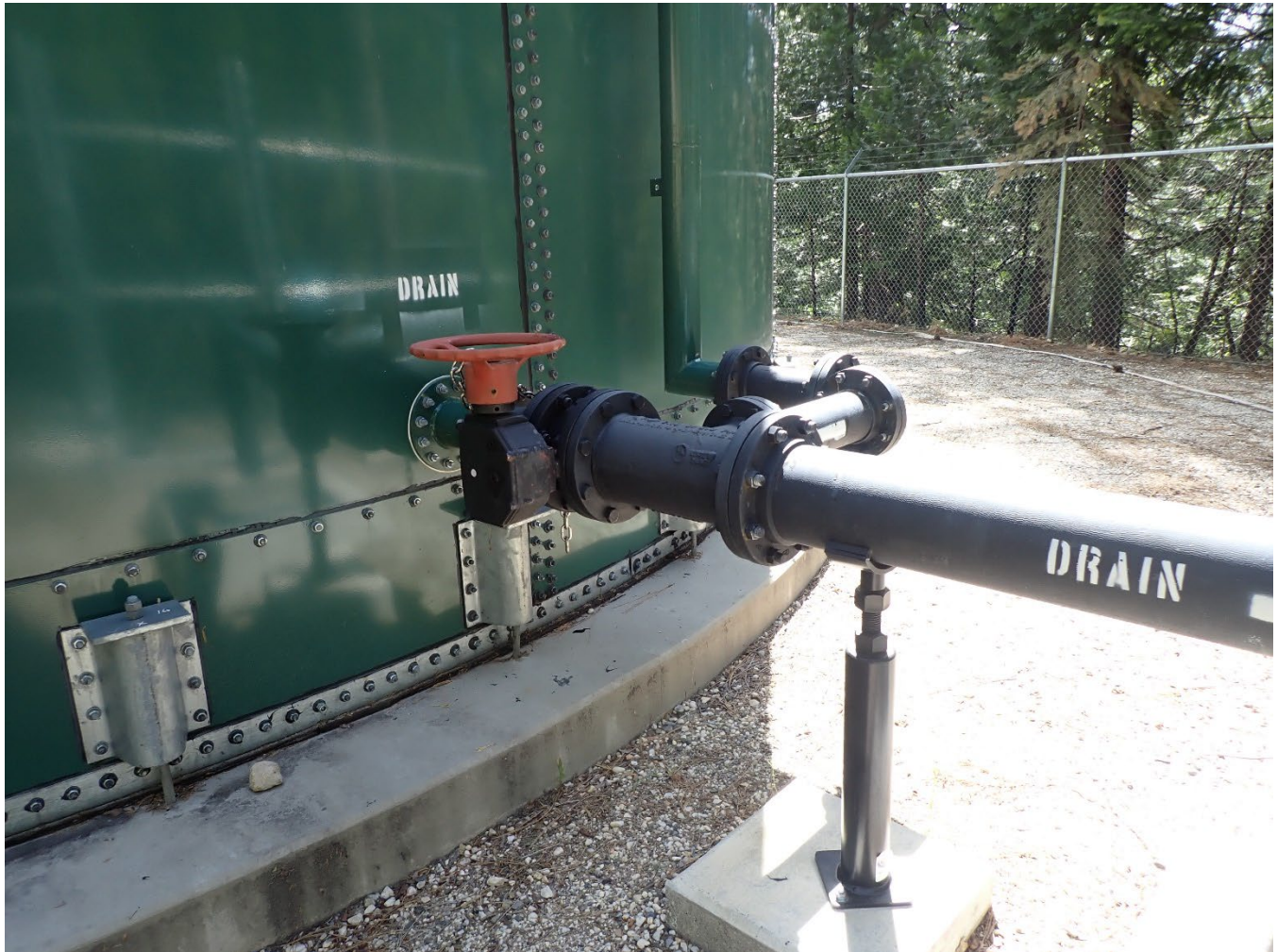
Exterior of the tank
