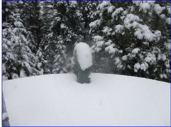
Photo 7 – Exterior (Jan 2020) – View of perimeter roof vent.
