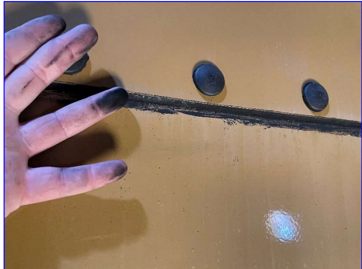
Photo 37 – Interior (June 2022) – View of residue wiped from the surfaces of the sealant.
