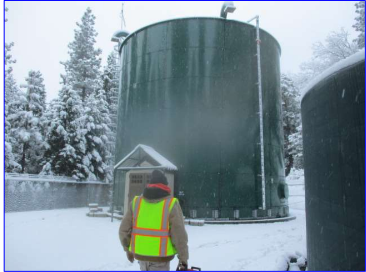
Photo 1 – Exterior (Jan 2020) – Overview of the Allegheny Bolted Tank
