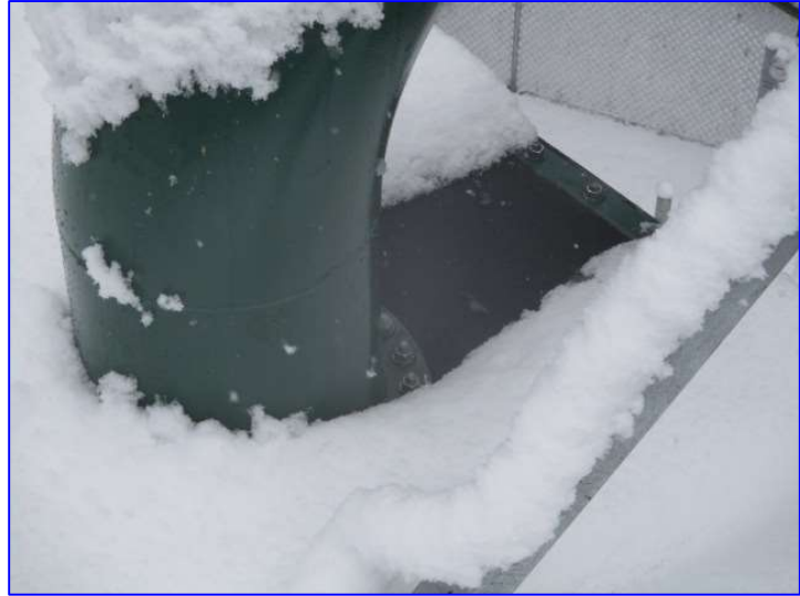
Photo 10 – Exterior (Jan 2020) – View of tank accessories.
