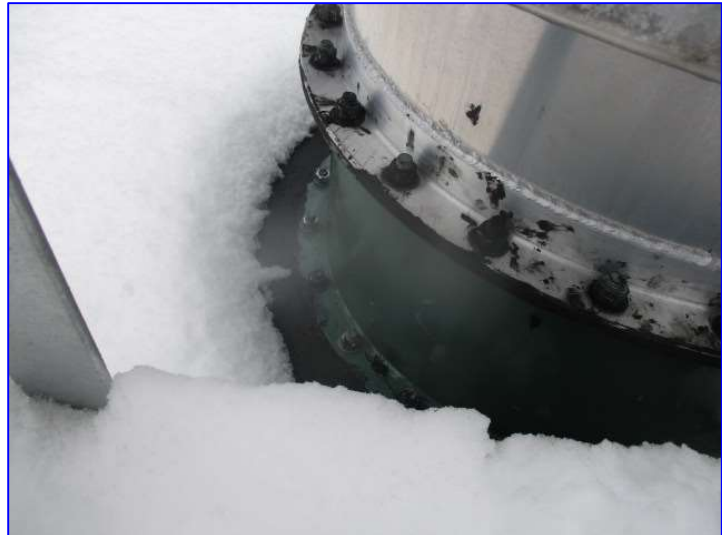
Photo 8 – Exterior (Jan 2020) – View of the aluminum center vent.
