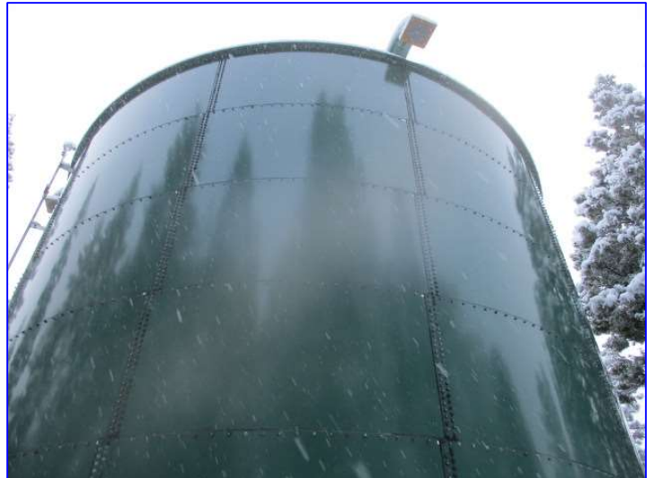
Photo 2 – Exterior (Jan 2020) – View of the six shell courses.
