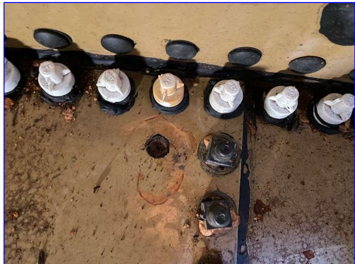
Photo 38 – Interior (June 2022) – View of a through penetration of the tank bottom.
