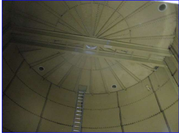
Photo 13 – Interior (Jan 2020) – Overview of the bridge supported roof structure.
