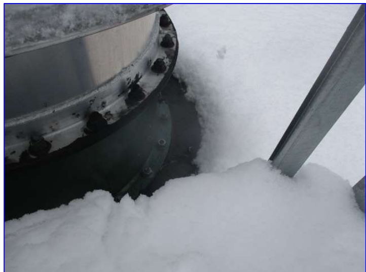
Photo 9 – Exterior (Jan 2020) – View of the roof center vent.
